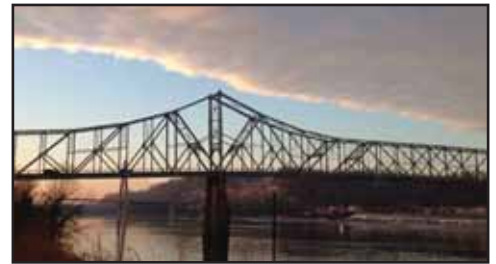
Ironton Russell Bridge
